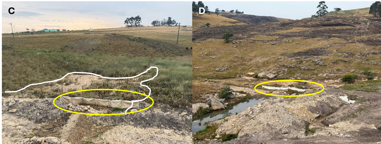
Figure 5 A) A sediment control structure that is completely ineffective or was installed after the sedimentation event occurred as indicated by the white lines. B) Is the downstream portion of the river channel that has been buried with sediment (CI number 11). C) A sediment control structure that has been completely bypassed by sediment washed from the road works and is now sitting within a wetland (CI number 2). D) A sediment control structure that has been completely bypassed by sediment washed from the road works and is now sitting within a river channel (CI number 6). Find coordinates of all photographs in Appendix A.
