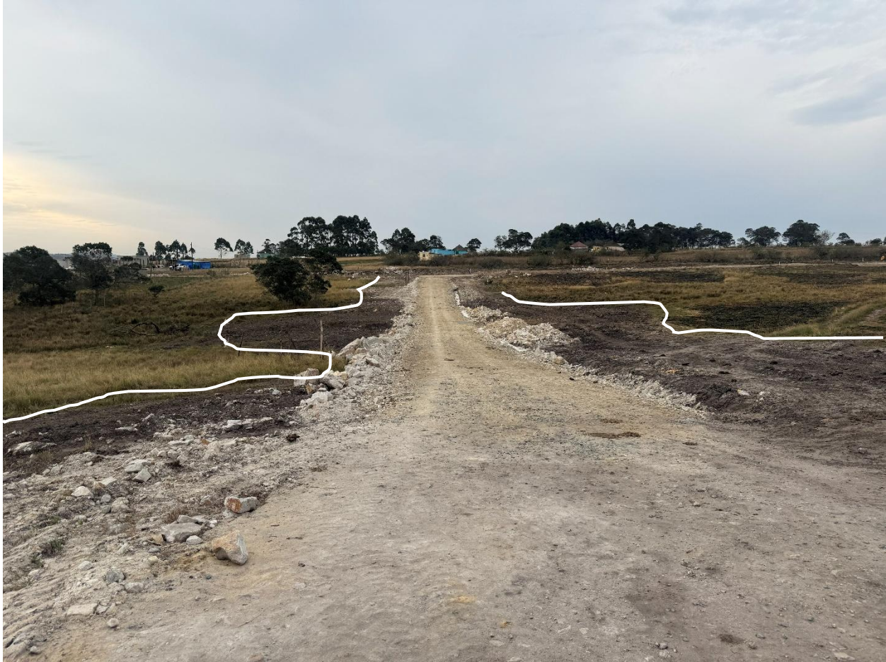
Figure 13 Road crossing through the head of a wetland. The road crossing appears to lead to a household and has no clear link to the N2 Road Construction site. Find coordinates of all photographs in Appendix A.
